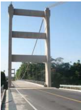
Bridge in Puerto Napo
